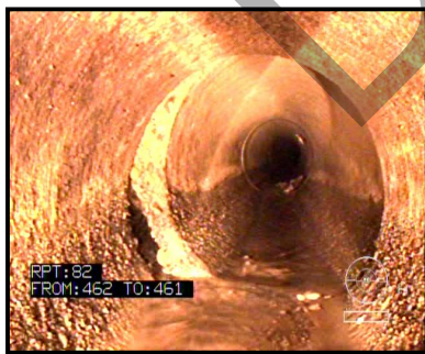
Figure 3.1: Medium Joint Displacement with voiding MH 462 to MH 461
