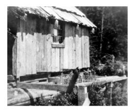
*Fig 2 "The Cabin"* (1932) Note the board and batten design with typical cedar shake roof and yellow cedar base log. This cabin was built from wood scavenged from the Nasmyth mill flume. (Gerry Harman Collection)
