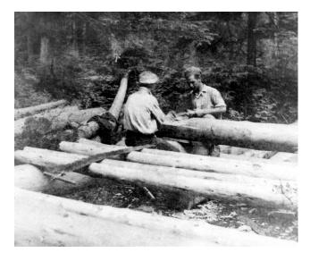
*Fig 7* Making a joint. These are flor strings that the saw is on (A. Charboneau collection 1936)
