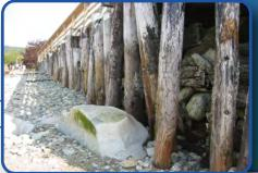
As waves hit the beach at an angle sediments are not just moved back and forth, instead they are gradually swept laterally, to the end of the beach and out to sea. Preventing this erosion from occuring safeguards shoreline structures and developments, as well as the beach. Boulders can be used to control the flow of water and sediments along the shore.
