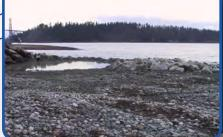
In 1965 due to concerns about erosion, sediments were dredged from the Capilano River and used to replenish Ambleside beach. Artificial beach nourishment is a temporary solution, however restoring the shore line to a more natural state would create a self-sustaining shoreline and improve the existing fish habitat.
