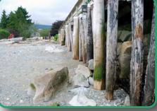
Tombolas are patches of boulders which guide and trap fine sediments carried by waves and currents. By retaining and stabilizing sediments in this way, we are able to use tombolas to increase the beach profile using natural coastal processes and provide long term prevention of beach erosion. Tombolas also act as wave trips and create intertidal habitat for rockweed, barnacles and mussels.
