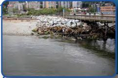
Ambleside has a wide, sloping stretch of sandy beach which is popular with visitors to the Seawalk. Without protection this stretch of beach is vulnerable to erosion by waves and longshore drift (the process by which waves and currents move sediments laterally along a beach), resulting in a heavily eroded beach to the west and infillling of the embayment to the east.
