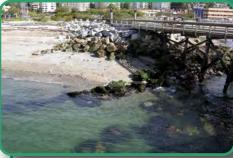
Rocks from the top of the riprap slope were reclaimed to create drift sills running along the the lower shore. Drift sills create a stable 'toe' at Ambleside Pier; interrupting longshore drift, disrupting wave energy and stabilizing the sandy beach at Ambleside along the beach stretching westerly to Lawson Pier. By working with natural coastal processes they provide a long term, sustainable solution to erosion.
