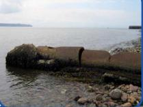
The two reinforced cement culverts exposed on the foreshore at 15th Street were badly damaged and eroded. Culverts and creeks are an important source of fine sediments for the upper shore and freshwater for many intertidal species. By removing the culvert pipes the fresh water and sediments could be retained on the upper- and mid-shore.
