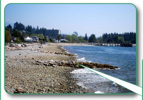
Boulders were strategically positioned to create tombolas and wave trips. Working like a natural rocky shore they 'trip' waves lower down the shore, and trap sediments along the upper shore, preventing erosion and encouraging natural beach replenishment. By working with natural coastal processes, wave trips and tombolas have long term benefits.
