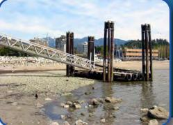
Ambleside Pier is a popular recreation site with public floats and boat launch facilities. Much of the fine sediment that was eroded from the beaches to the west of the pier was deposited in this sheltered cove. As the sediment infill accumulated it reduced the depth of the cove; during low water the boat launch was unusable and the public float was almost entirely stranded.
