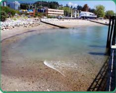
The area between the boat launch and public float was dredged to remove the sediment infill, allowing boats to be launched and safe water access to the public float at all times. The drift sills created to the west of the pier will reduce the rate of sediment infill in the future, providing ongoing protection for the boat ramp and float.
