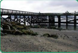
Boulders taken from the existing riprap slope were repositioned along the lower shore to make drift sills, creating a stable 'toe'. As longshore drift is interrupted, fine sediments are held in place on the shoreline and erosion is reduced. By working with natural processes, drift sills can provide long-term prevention of erosion and are environmentally sound.
