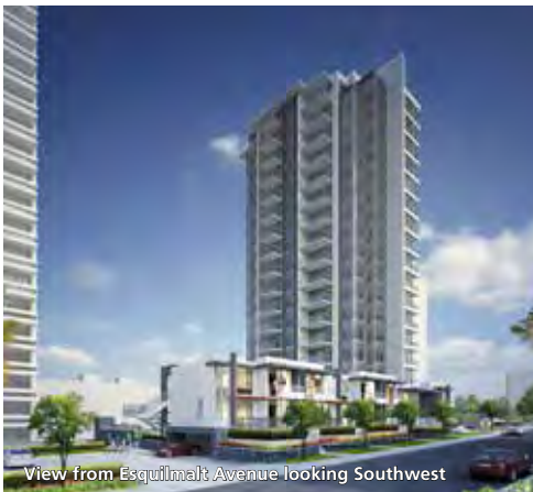
View from Esquimalt Avenue looking Southwest
