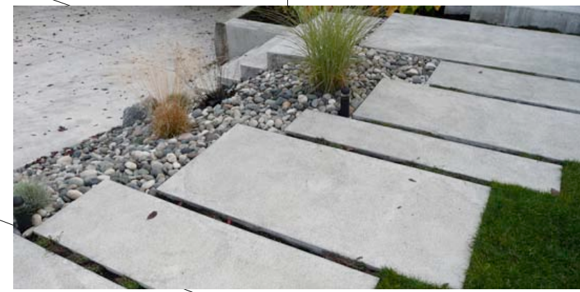
Cast in Place Concrete Stepping Stones
