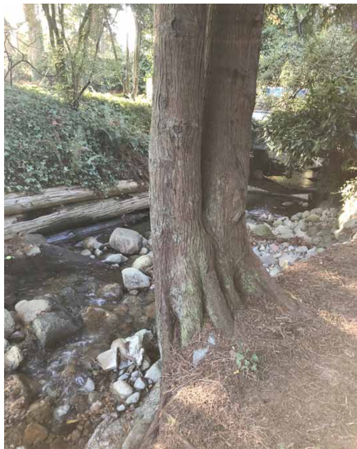
Base of Tree #41 along top-of-bank.
