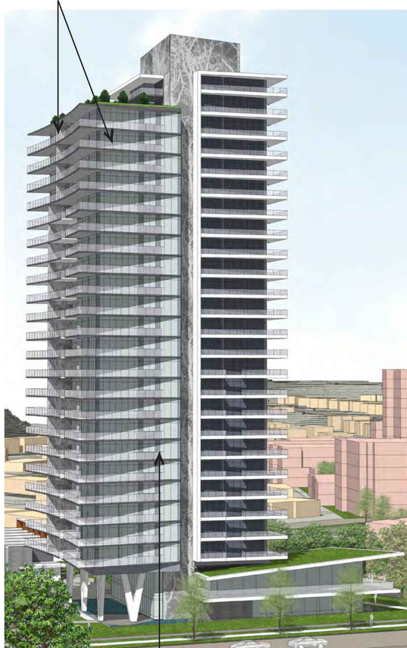
Concrete overhangs provide passive solar control
