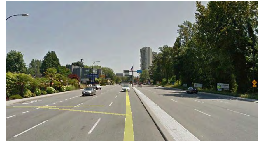
F MARINE DRIVE LOOKING EAST
