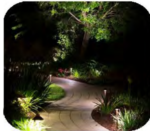
SHIELDED PATH LIGHTING
