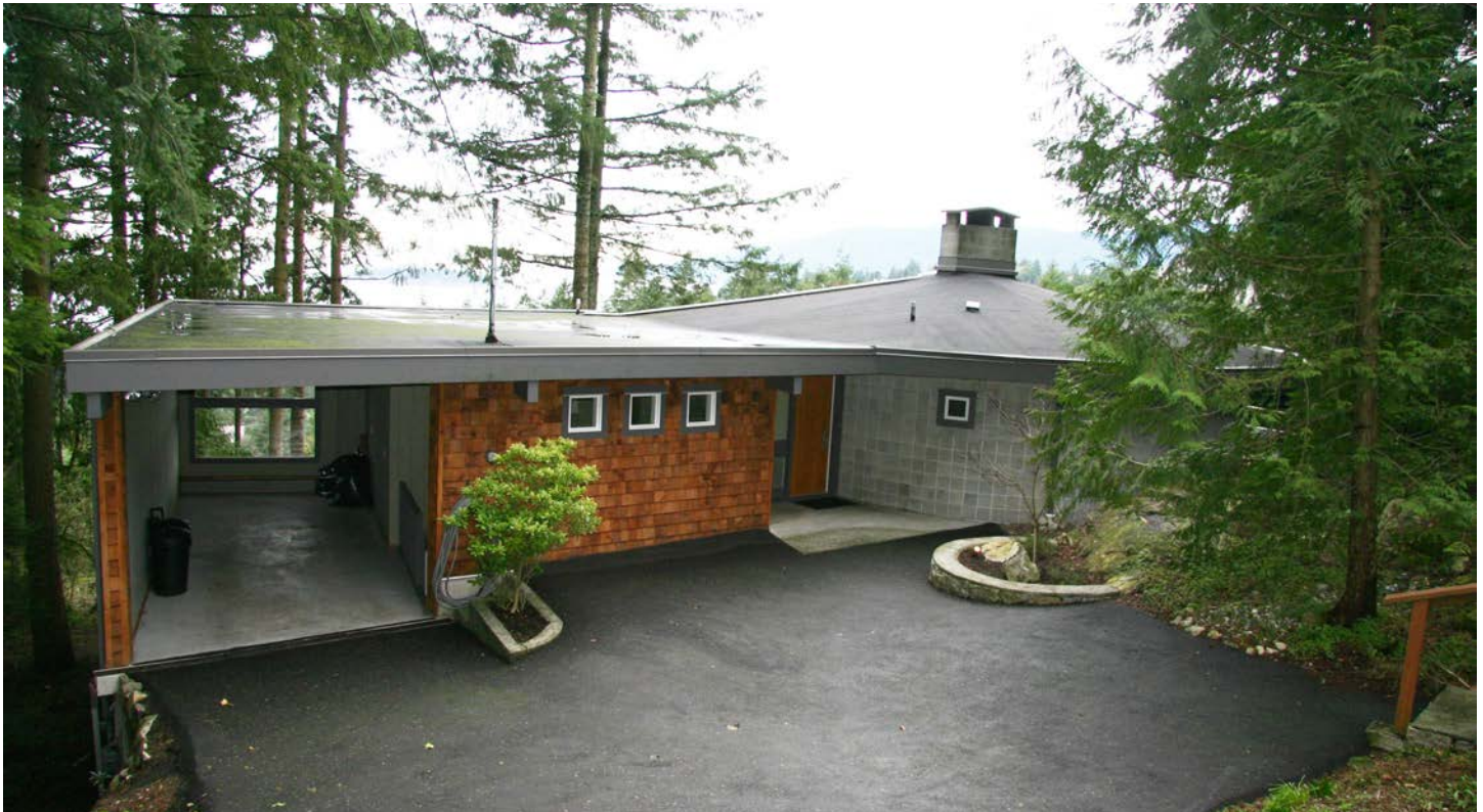
Flat roof above carport and office
