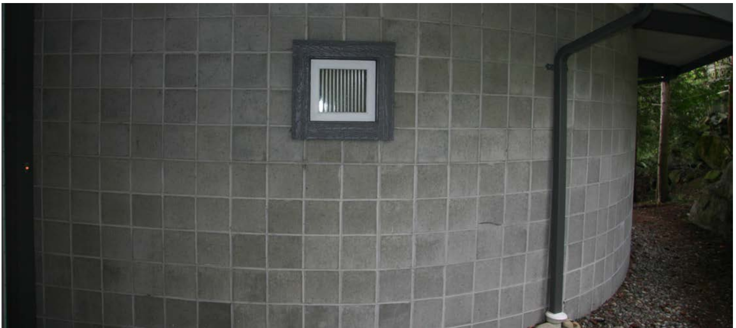
Original 'Denstone' block wall
