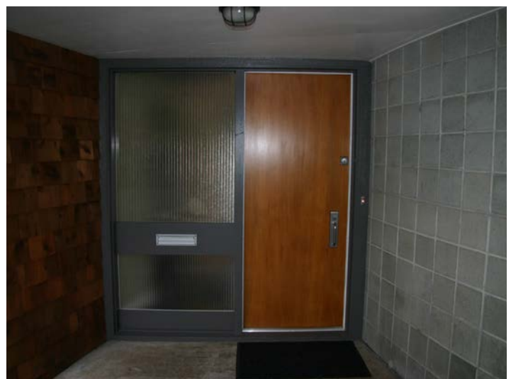
Original front door assembly with reeded sidelights
