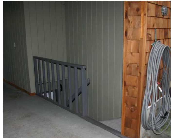
Carport walls finished with original wood siding
