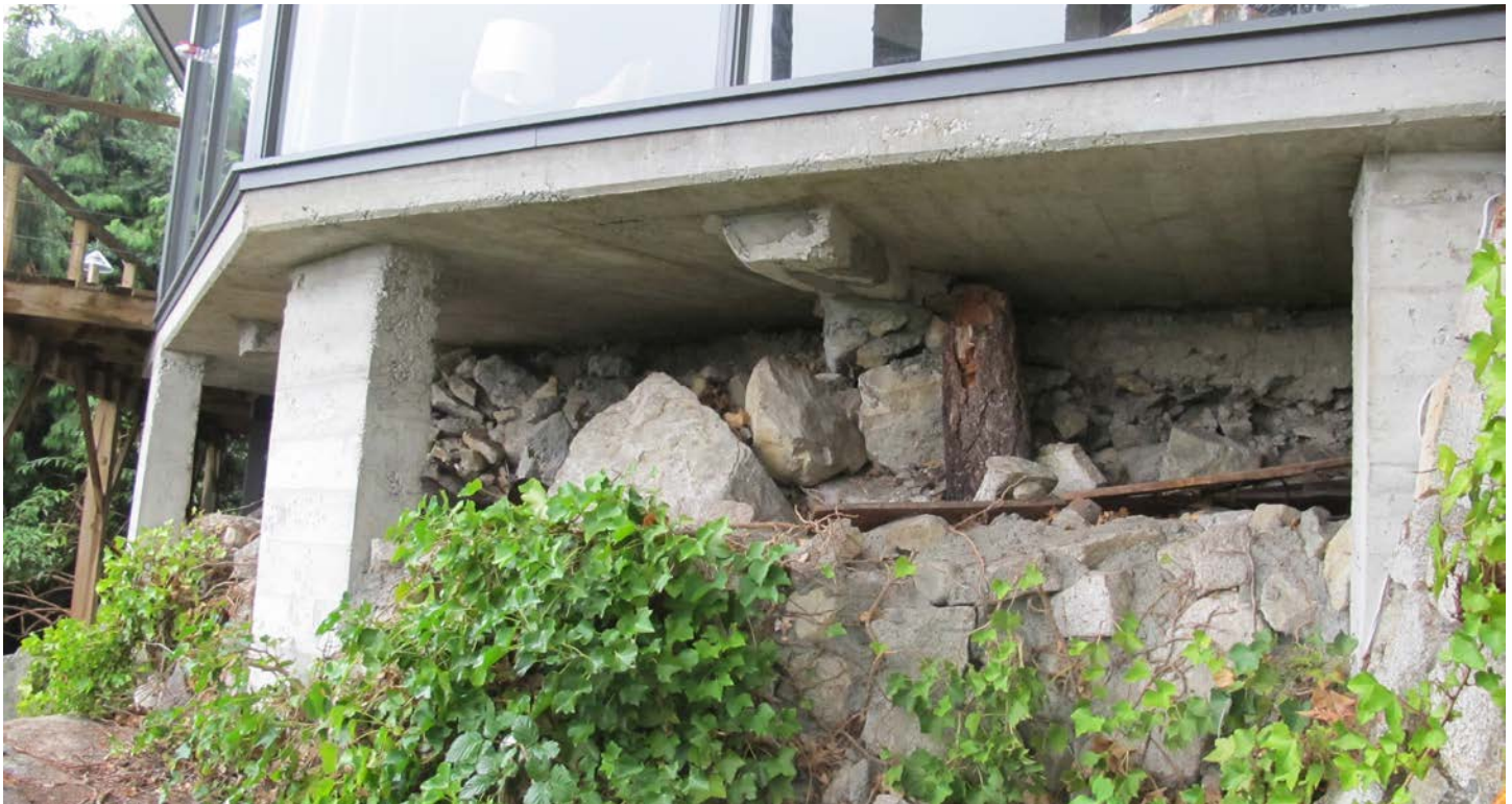
Concrete pillars support the cantilevered floor slab of the living room
