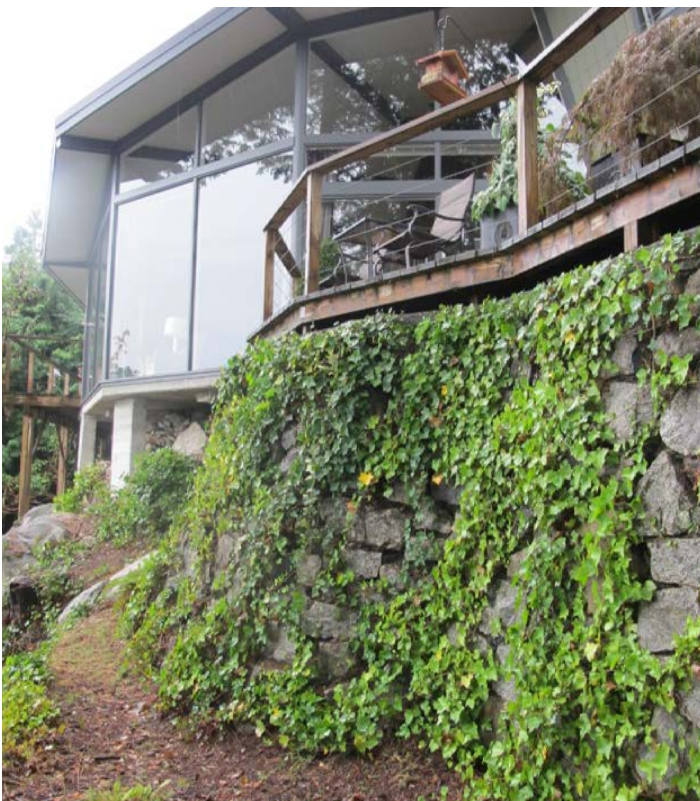
Granite retaining wall covered with ivy
