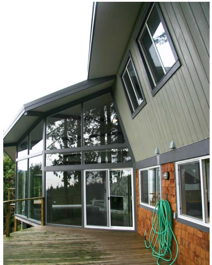
Angled upper wall with original wood siding, lower level with new cedar shingles
