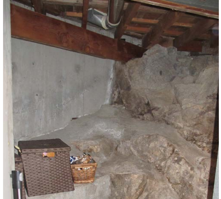
Concrete foundation wall built into bedrock
