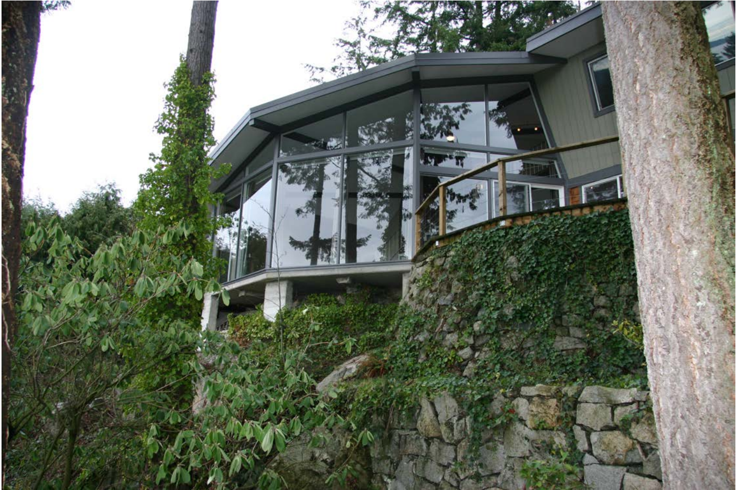
South view of the elevated Sykes Residence
