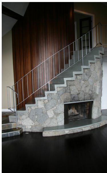
Concrete stair above granite-faced fireplace
