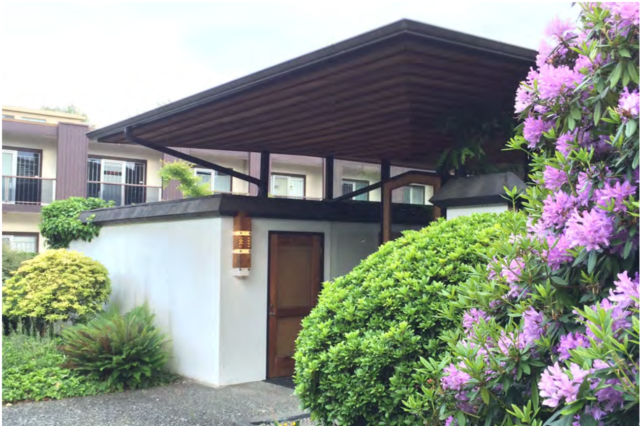
Below: The building in 2016
