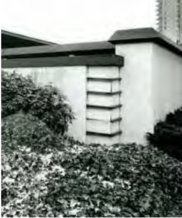
Cracked glass in the clerestory
