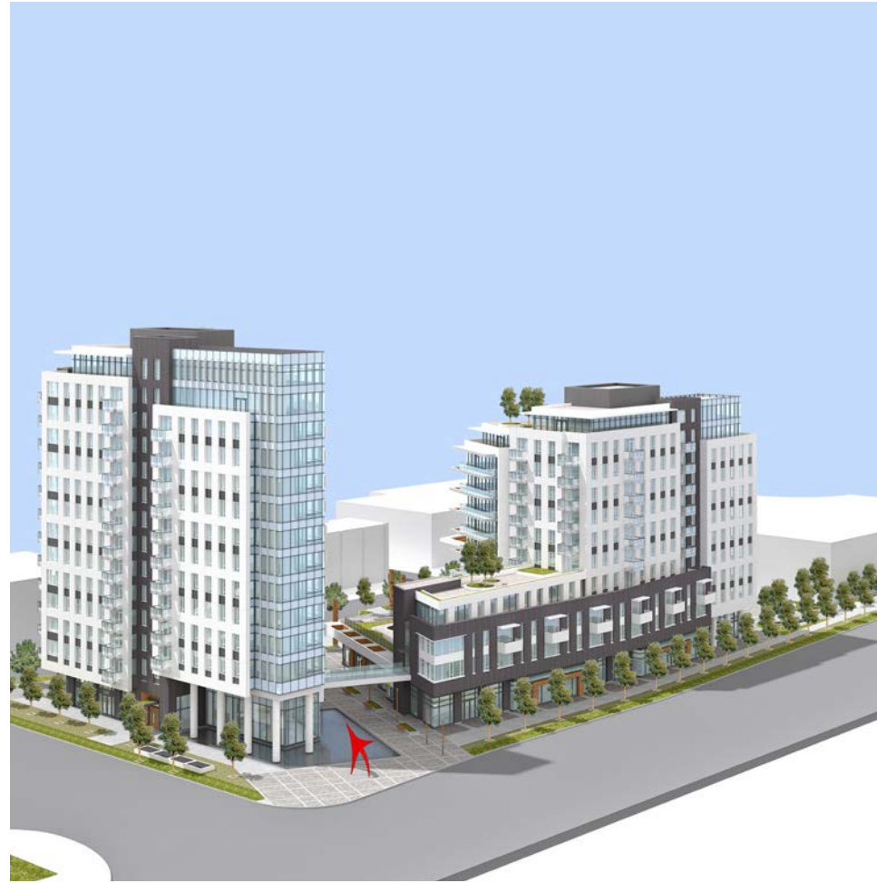
VIEW FROM NORTH EAST
