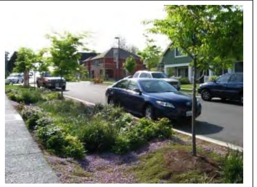
A Bioswale will handle water run off on Taylor Way.
