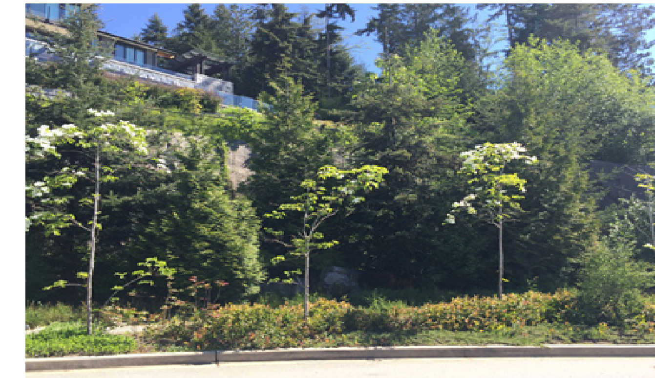
Shotcrete Wall (precedent image - several years after)
