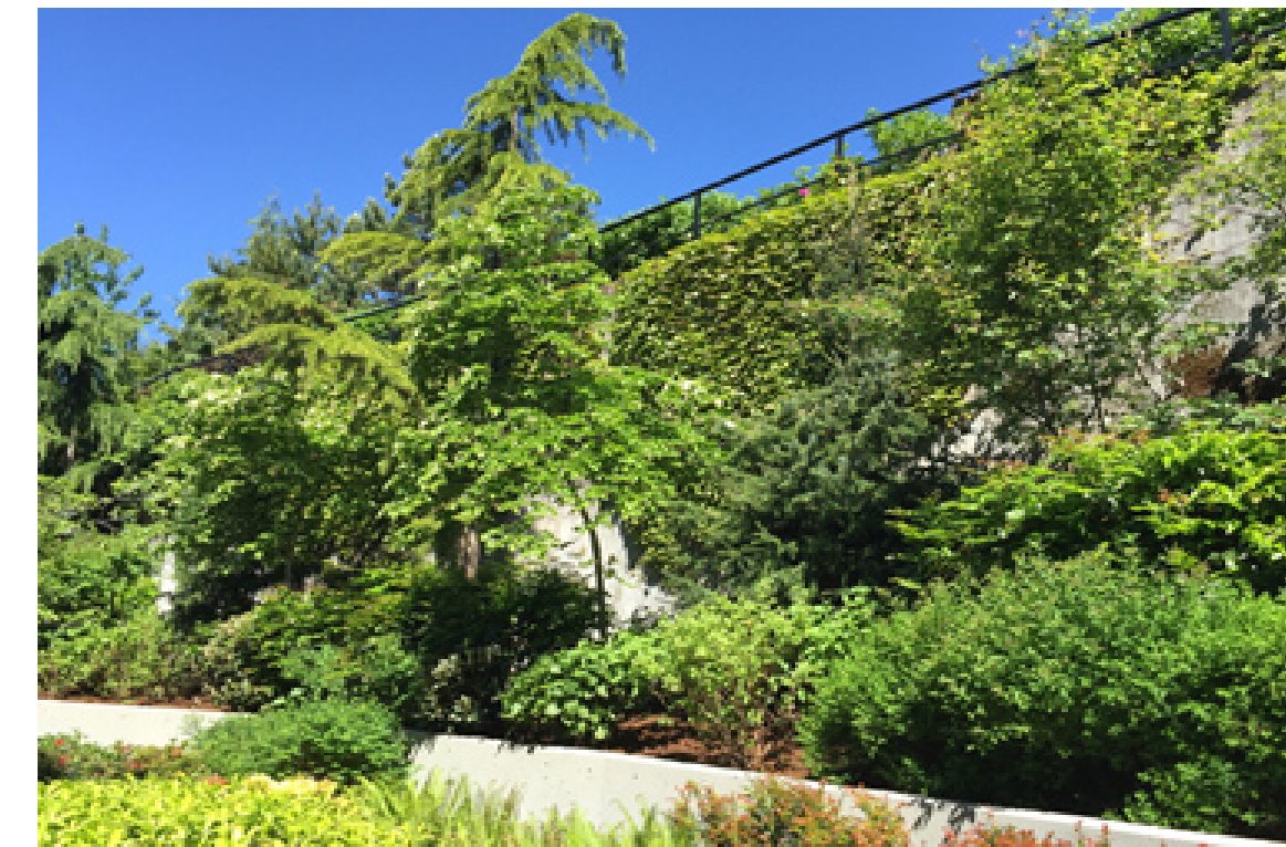
Shotcrete Wall (precedent image - several years after)
