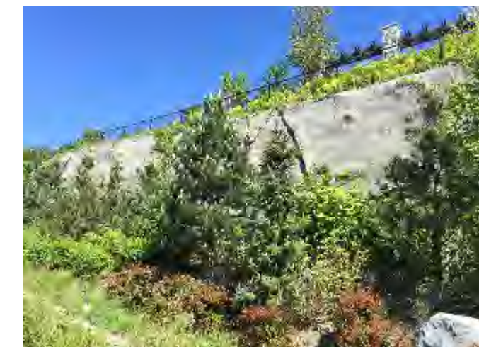
Shotcrete Wall (precedent image)
