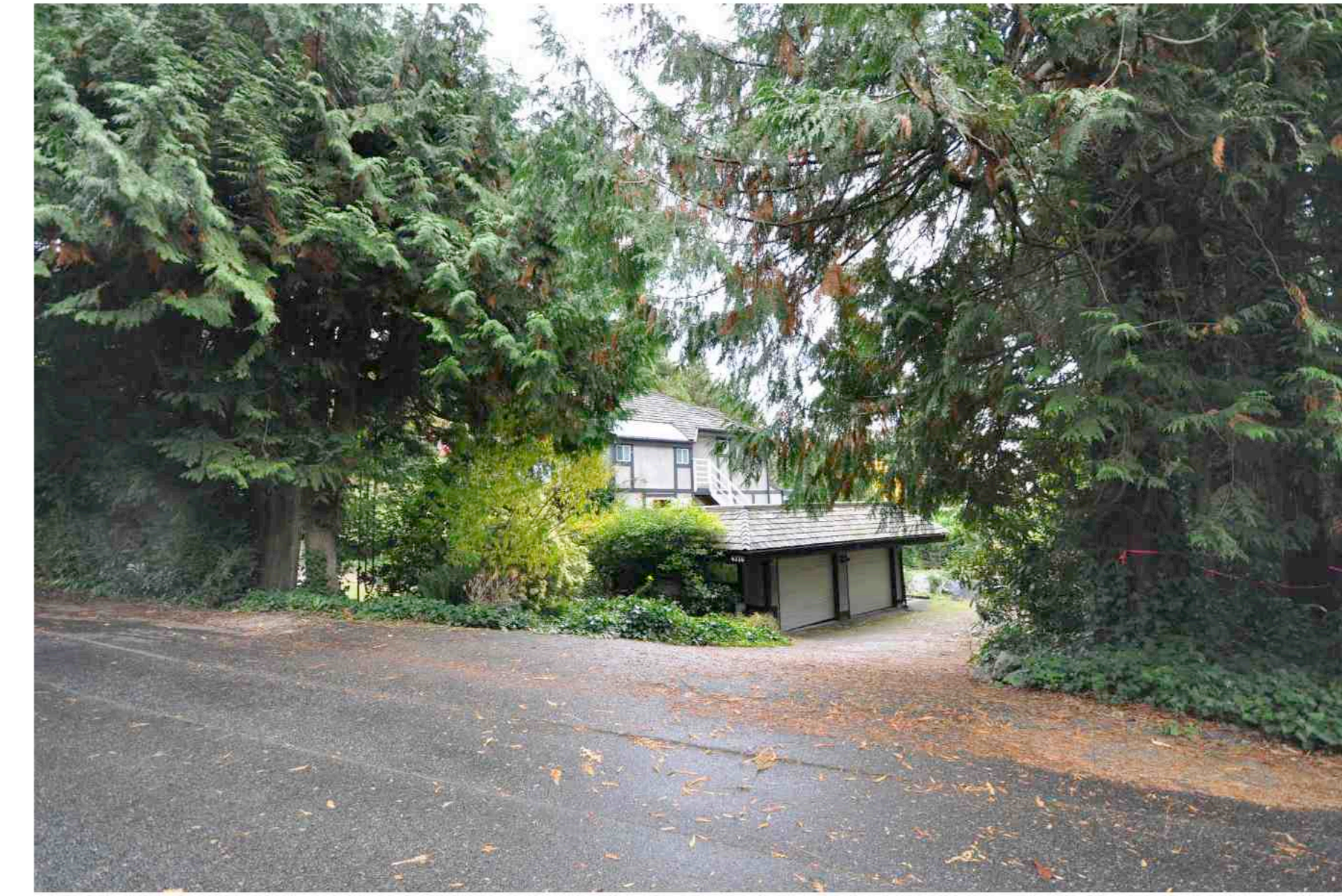
THE HIGHWAY ENTRY
