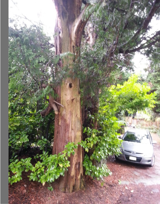
Photo 1: The subject tree has significant wounds on both trunks most likely from historic vehicle damage.
