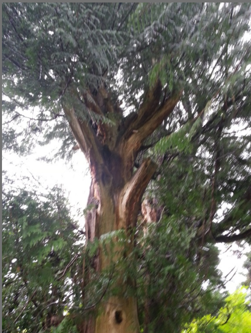
Photo 1: View of the very poor structural condition and the previously topped form of the subject tree. Note the necrotic bark extends from the base to into the top.
