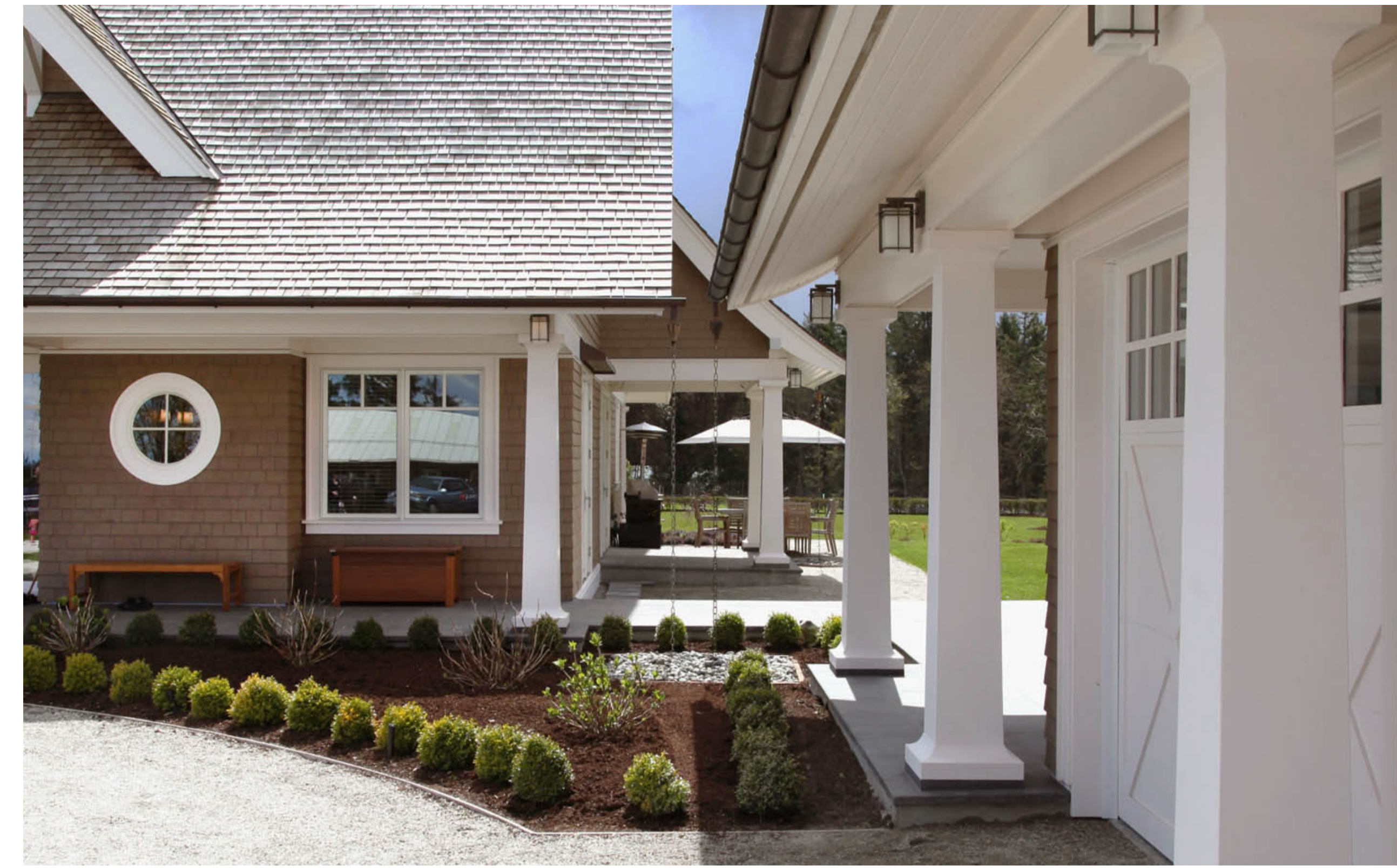
11 The materials, colours and textures of the exterior of the house will be reminiscent of the shingle-style craftsman houses built in West Vancouver a hundred years ago at the time lower Caulfeild was being developed. The columns, for example, will be in the rectangular form that carpenters built on site.
