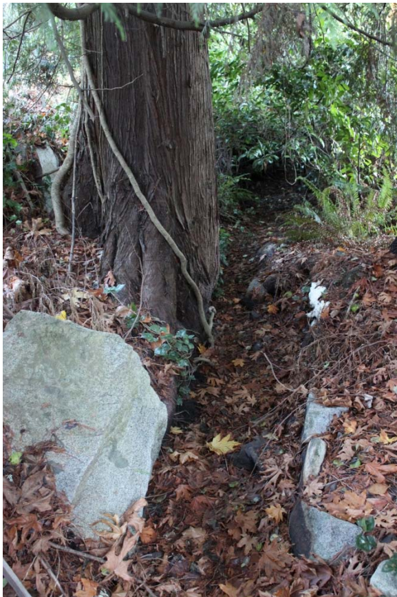
Photo 2. Manmade drainage channel running west to east along north boundary of property. View looking upstream (west).
