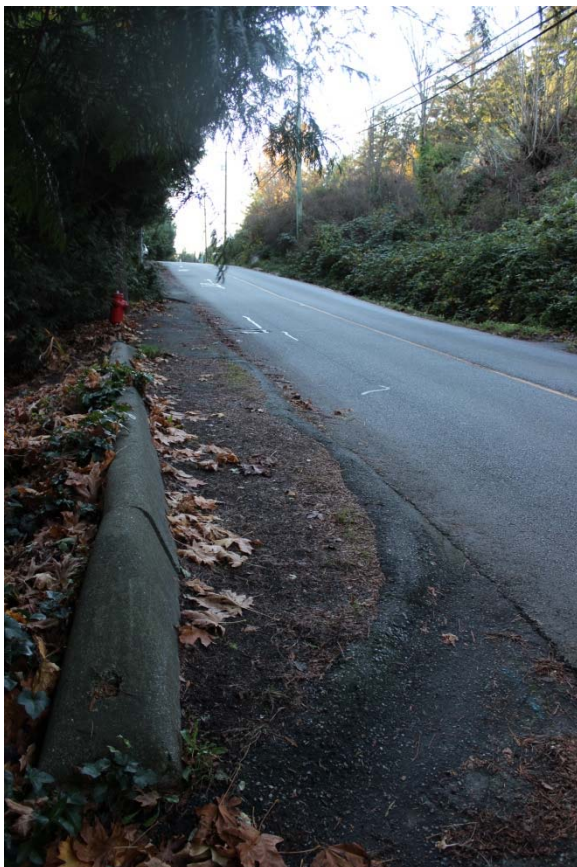
Photo 4. Road drainage from Marine Drive directed to drainage channel. View looking west on Marine Drive.
