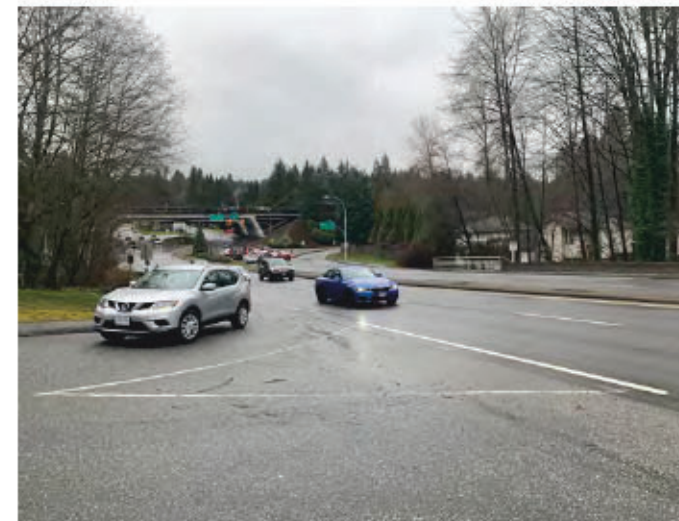
5 Right in, right out at north of site from Jewish Centre parking and fire lane.
