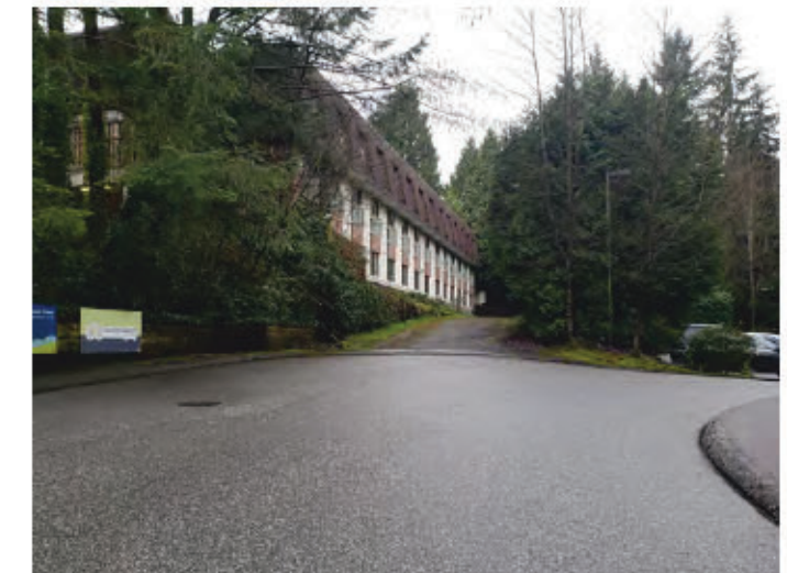
6 Fire lane at north of site.
