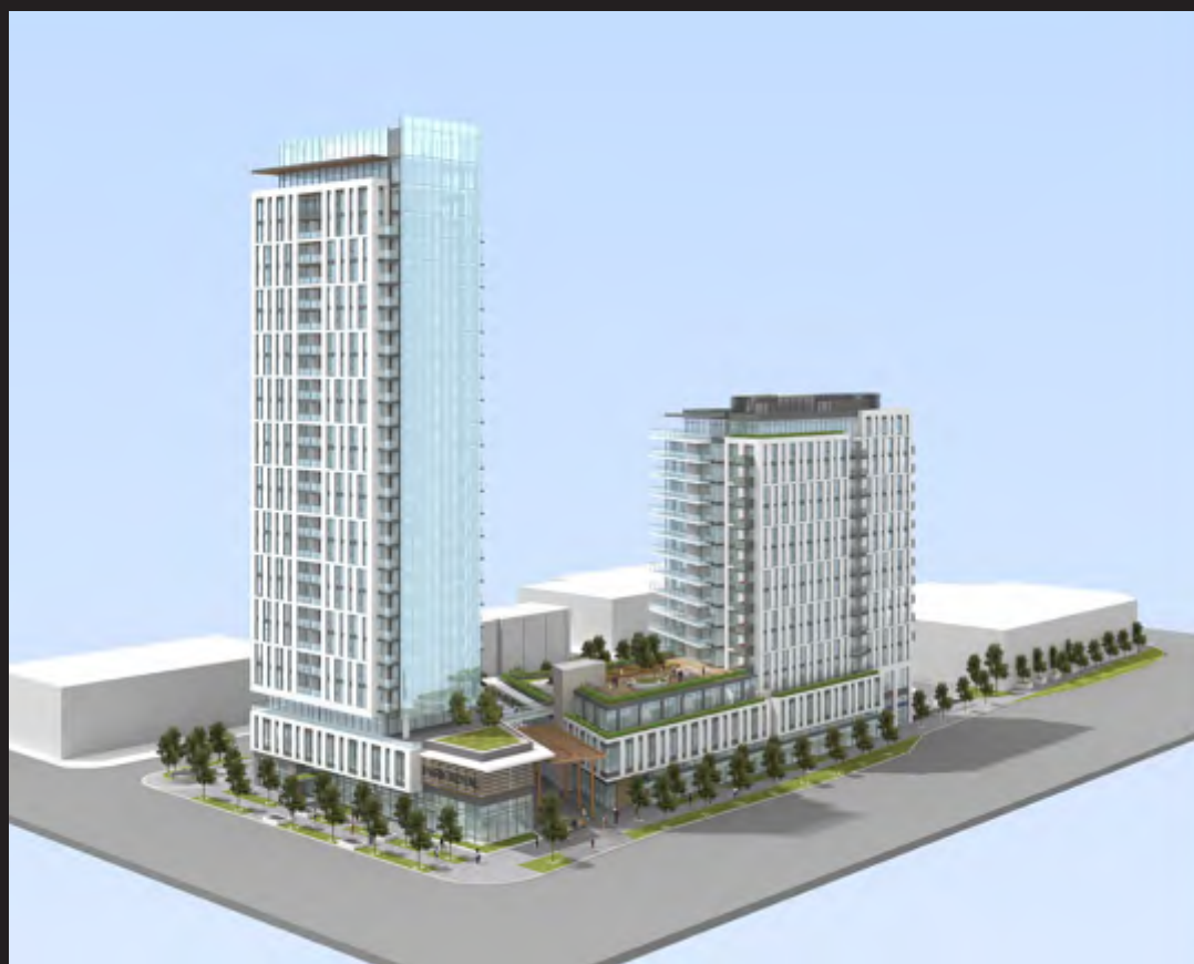
VIEW FROM NE
