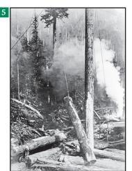
This site area was the upper terminus of a cable railway where logs were loaded on rail cars attached to the cable of a "snubbing" donkey and lowered to a shingle mill several kilometres below.
