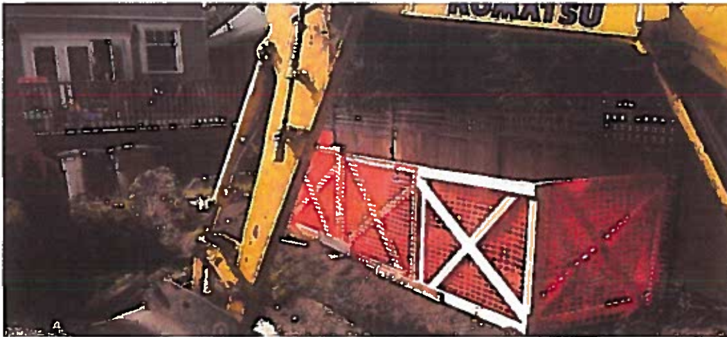
Tree fencing-wood framed snow fence
