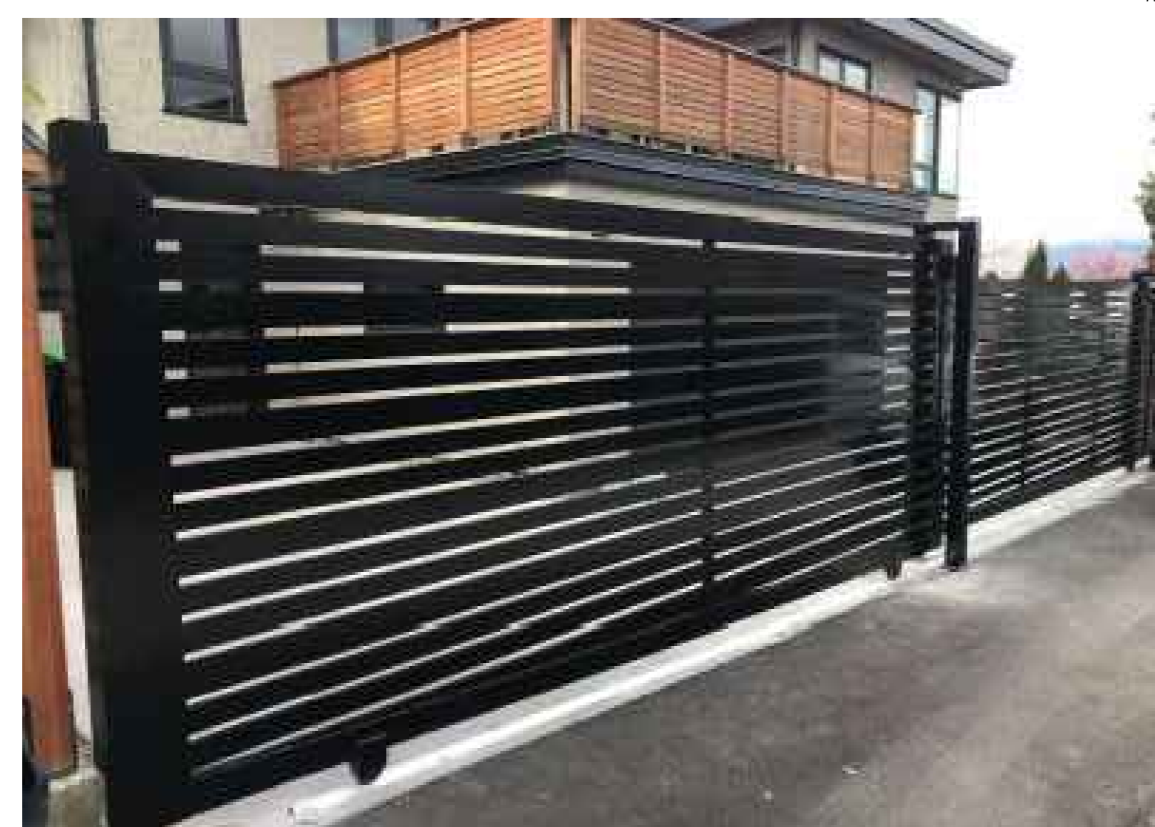
SLIDING GATE AT DRIVEWAY
