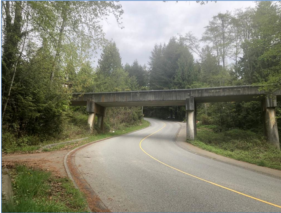
Figure 10: Existing Driveway on Westport Road - Looking north
