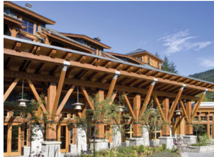
Village character - roof form and exposed structural elements
