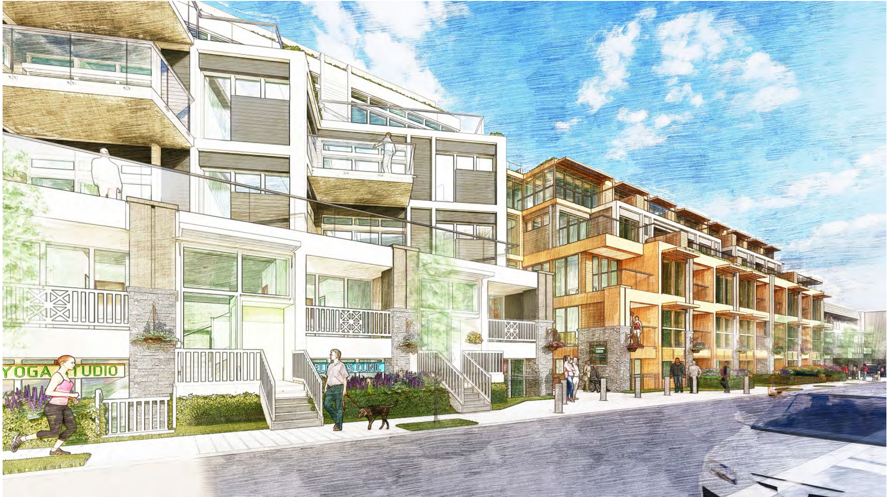
DUNDARAVE LANE - LOOKING NORTHEAST
