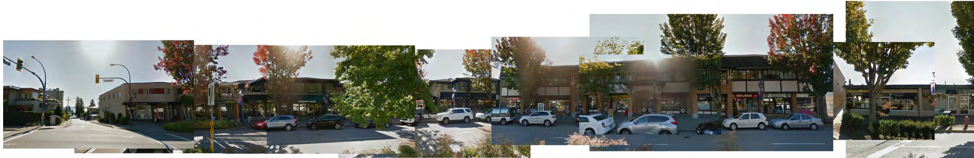
4. MARINE DRIVE (SOUTH) - FACING SITE
